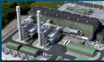
Electric Cabins & Substations
