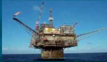
Platforms & PV Installations
